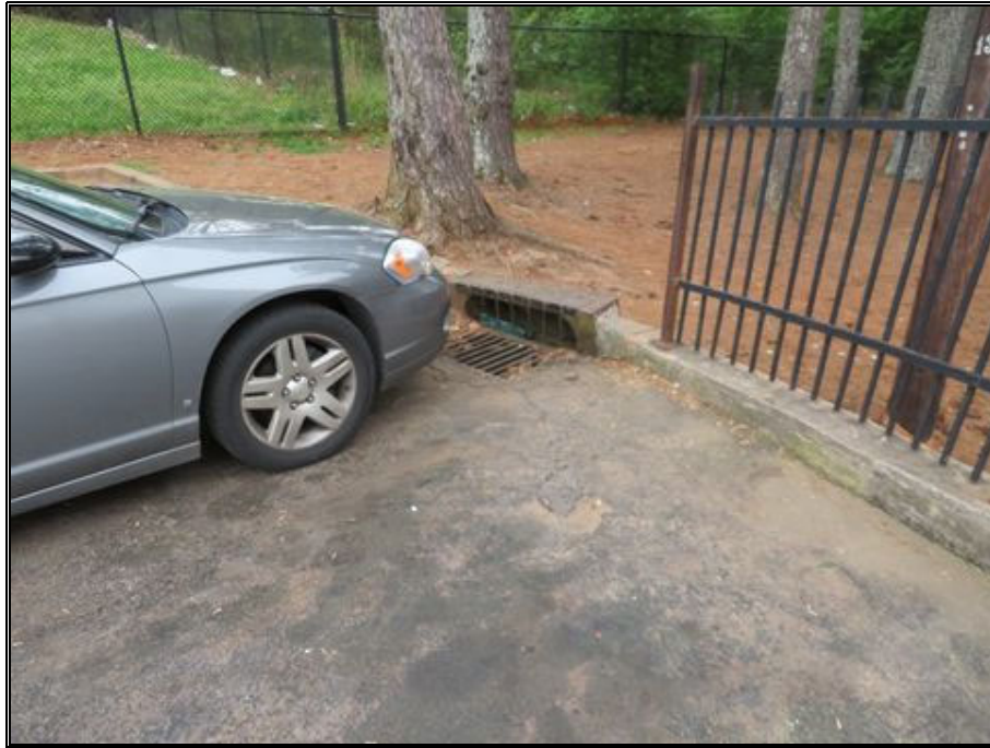
P37-Typical Upper Level Curb Drain
