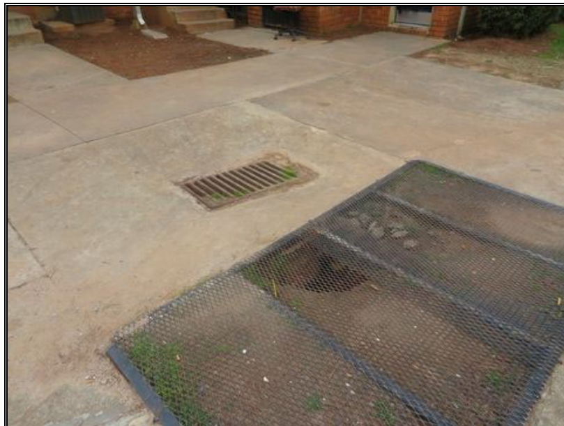
P8-Sidewalk Storm Water Drain
