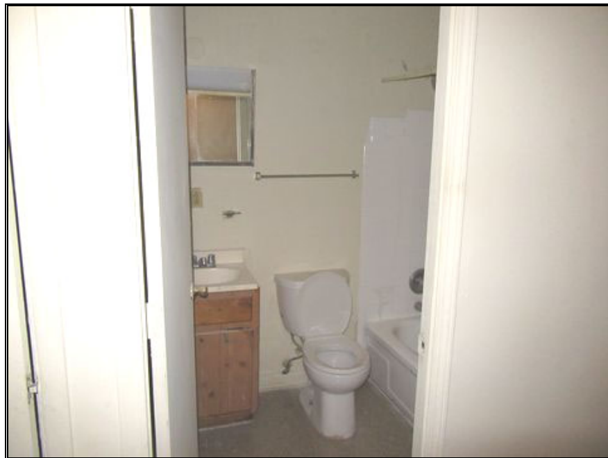
P62-Vacant Unit Bathroom
