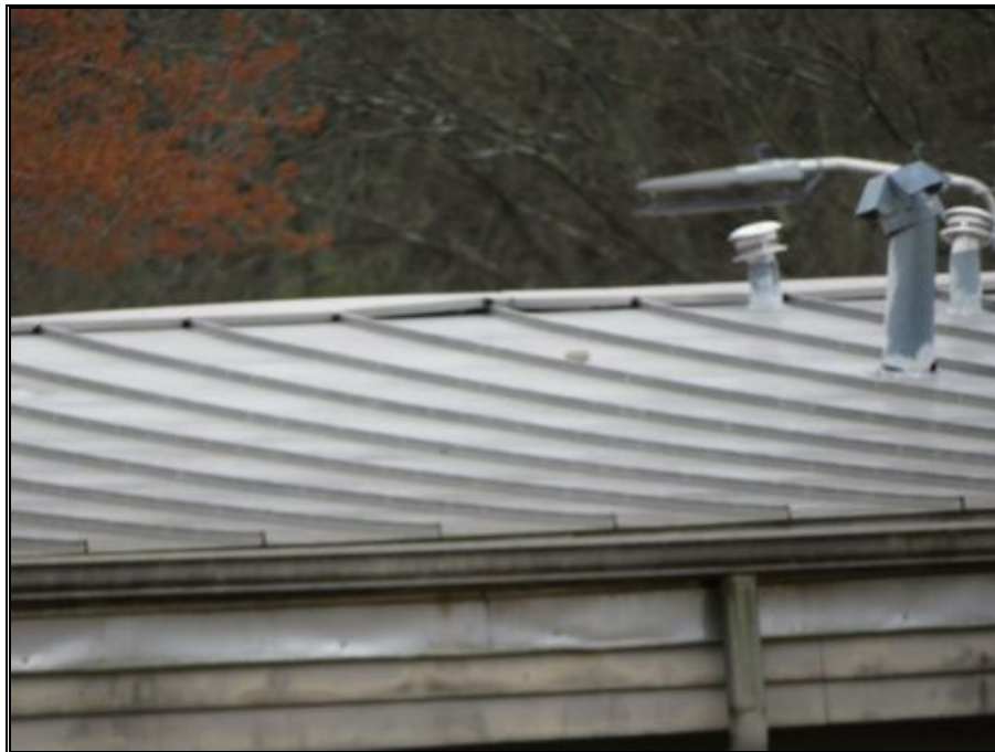
P34-Typical Steel Roof and Vents Condition
