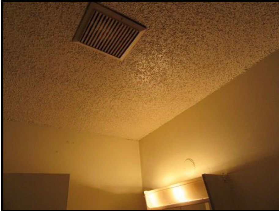
P75-Typical Bathroom Fan
