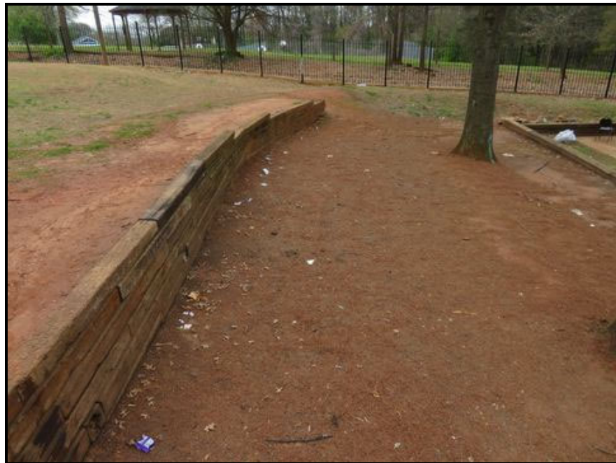
P54-Wood Retaining Wall
