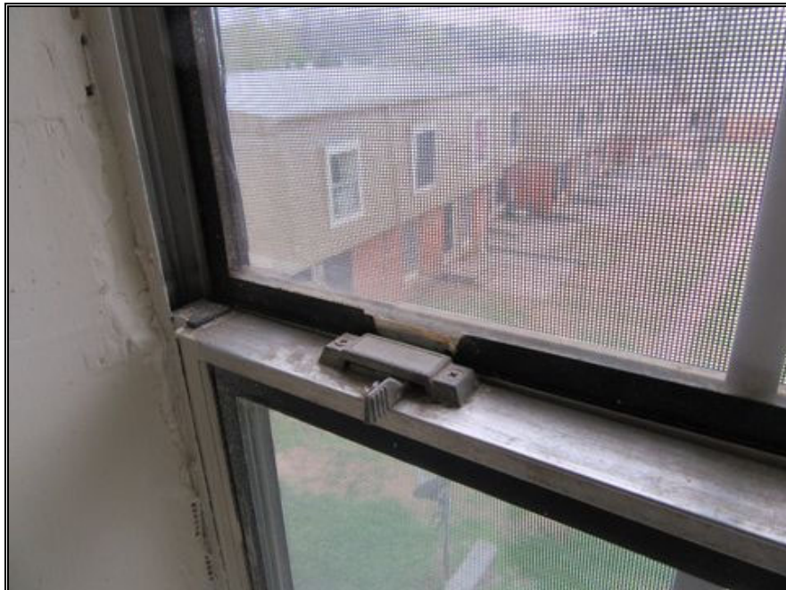
P68-Typical Window Condition
