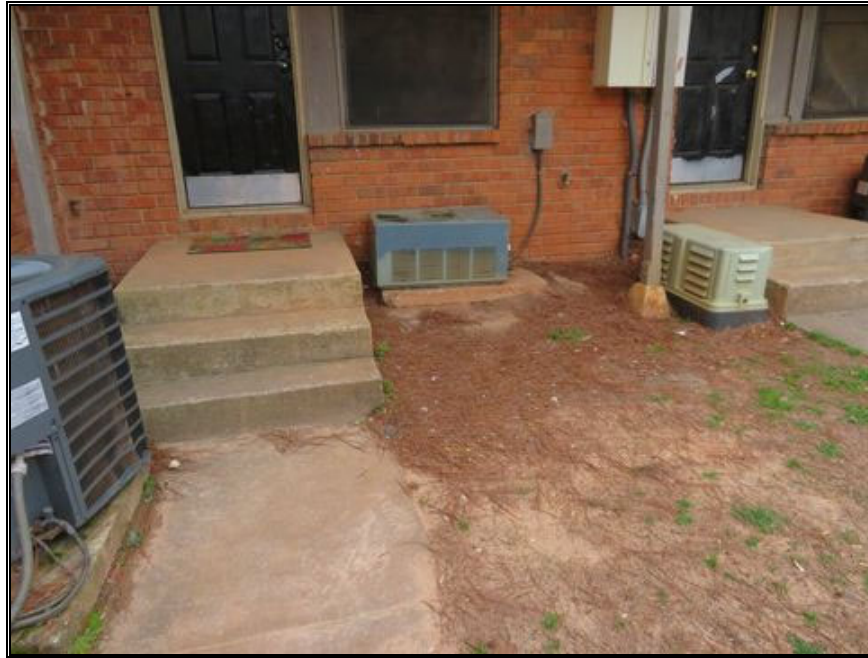
P29-Typical Air Condensers Variety
