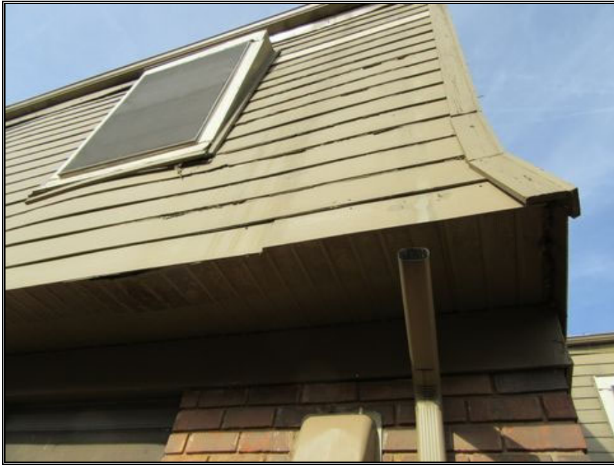
P89-Window Pulling Out of Frame
