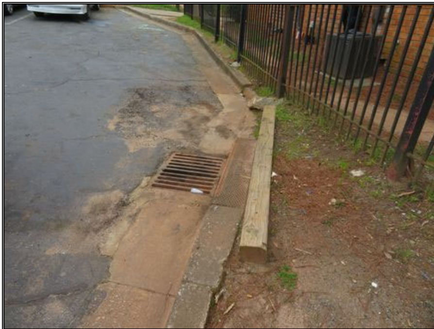
P24-Typical Condition of Curb Drains
