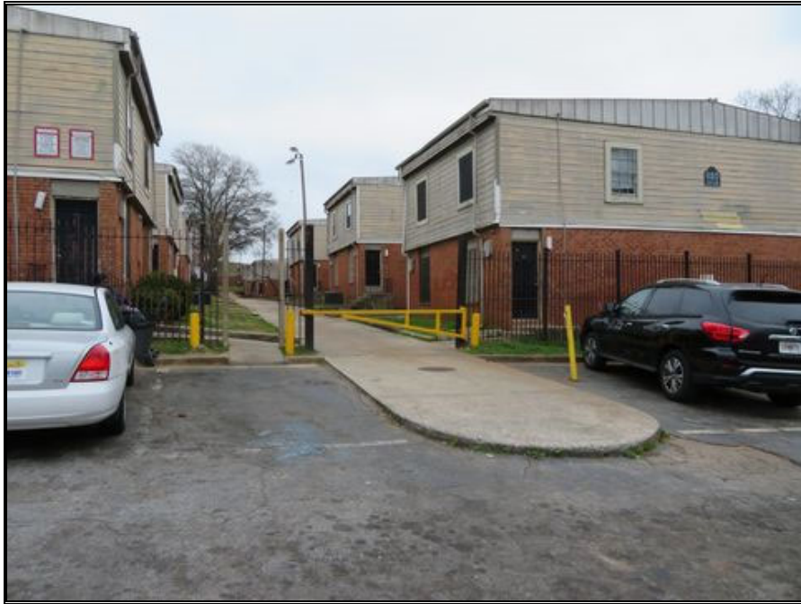
P25-Gate at Entrance between Buildings
