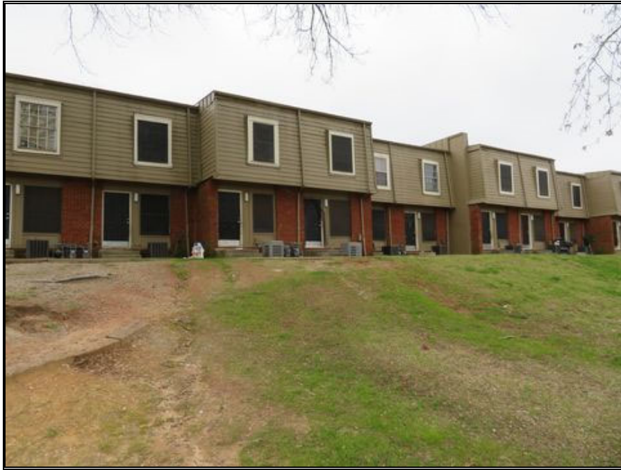
P51-Building Rear Elevation/Eroded Hillside
