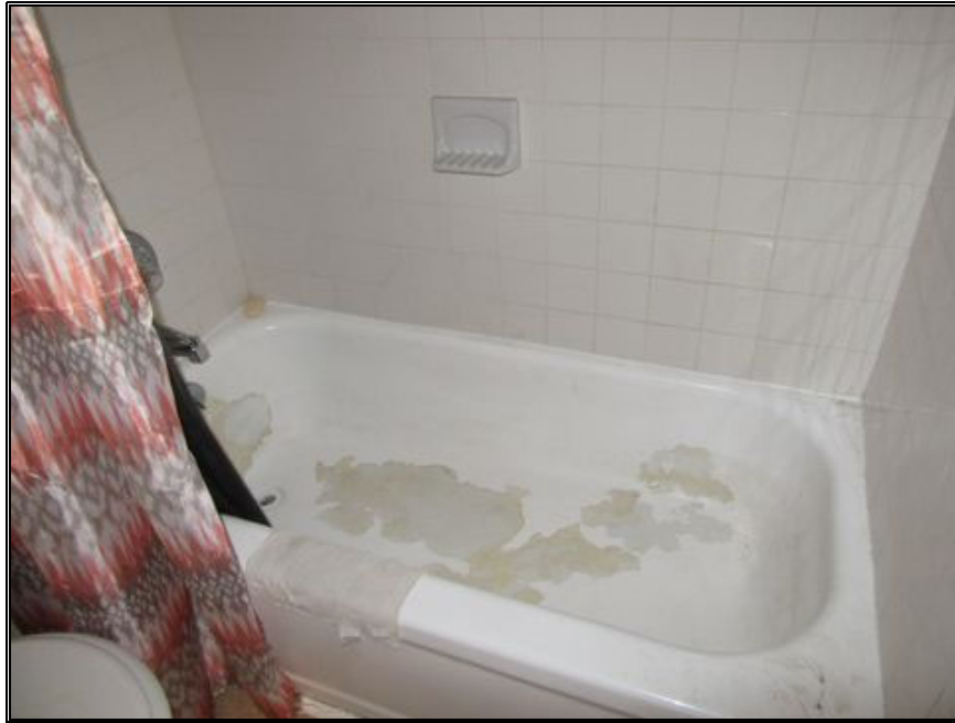
P83-Typical Poor Tub Condition
