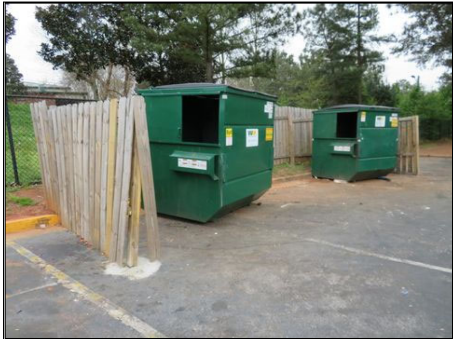
P36-Dumpster Area with Wood Surrounds in Fair to Poor Condition
