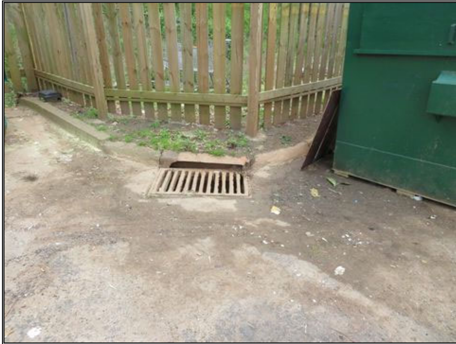
P15-Typical Curb Drain
