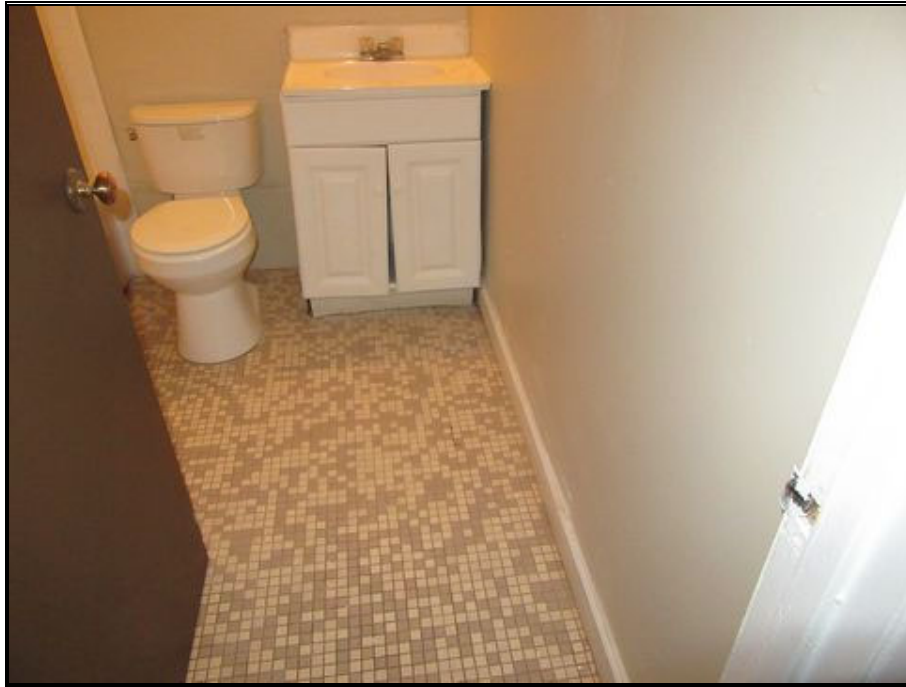
P71-Vacant Unit Bathroom (Poor Vanity)
