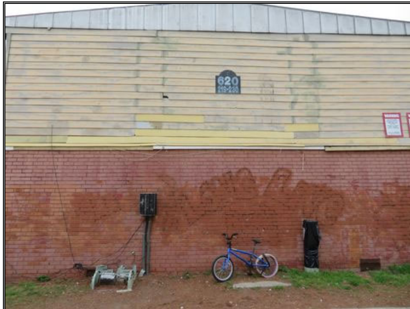
P18-Typical Condition of End Gable Areas
