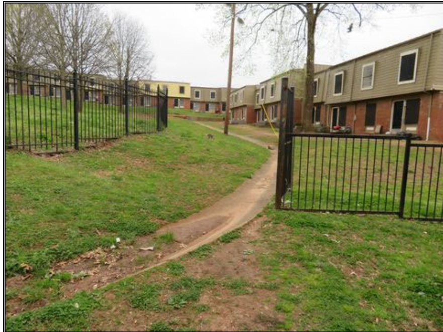
P26-Typical Concrete Sluceway for Storm Water
