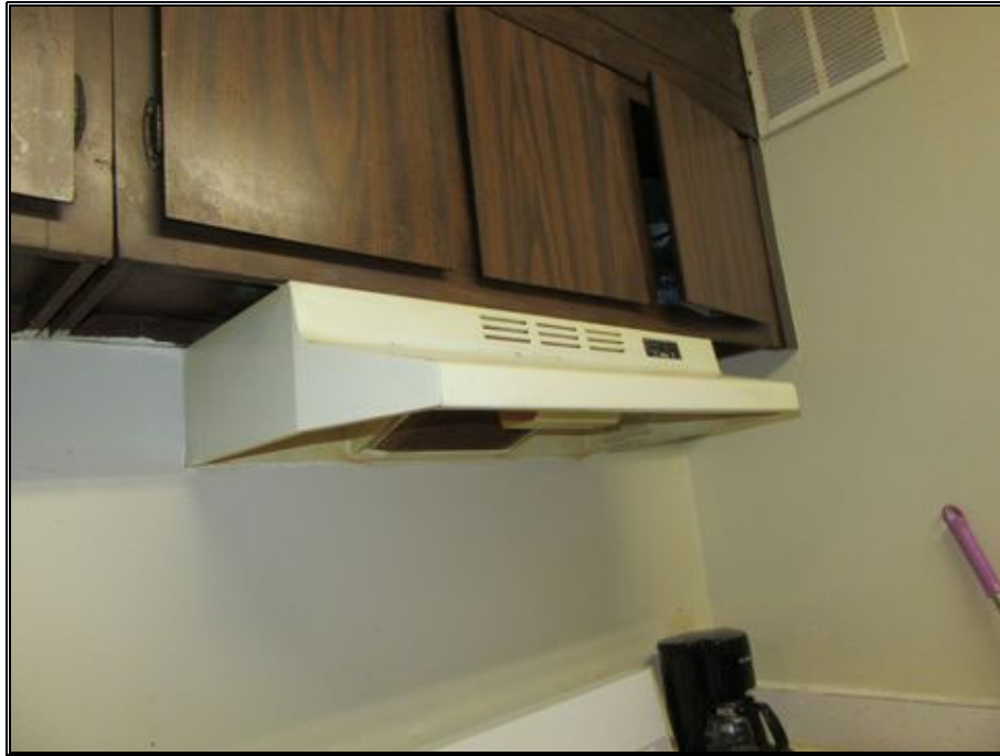
P79-Typical Re-Circulating Range Hood
