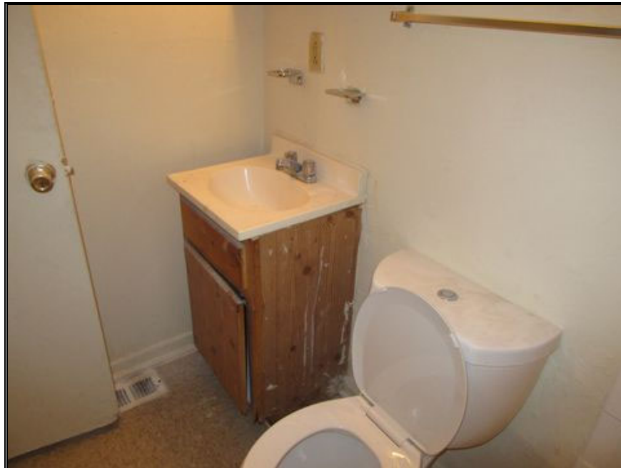
P64-Vanity in Poor Condition
