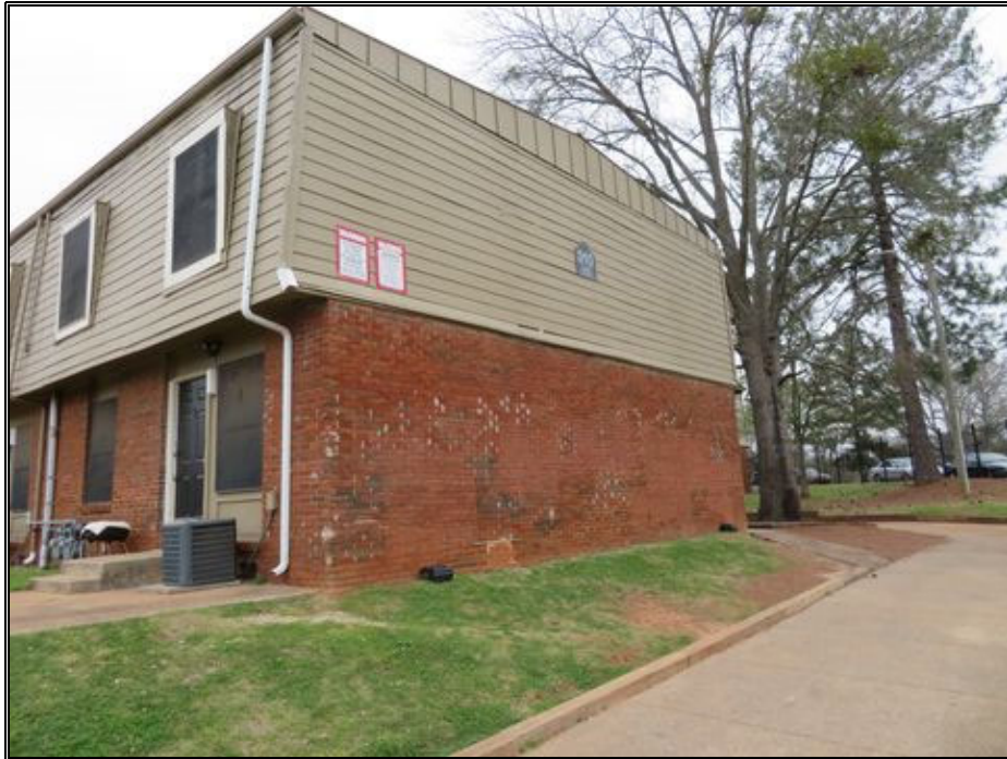
P39-Residential Building End Elevation Brick Condition
