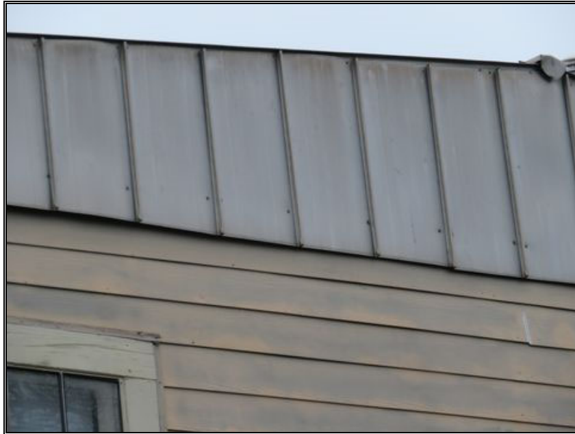
P17-Metal Gable Area
