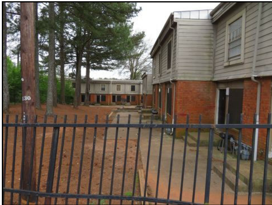
P38-Fence and Residential Buildings Rear Elevations
