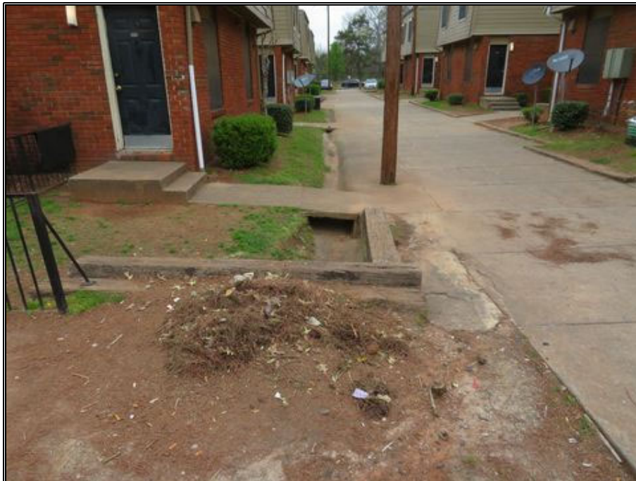
P50-Drainage Sluiceway in Front of Buildings
