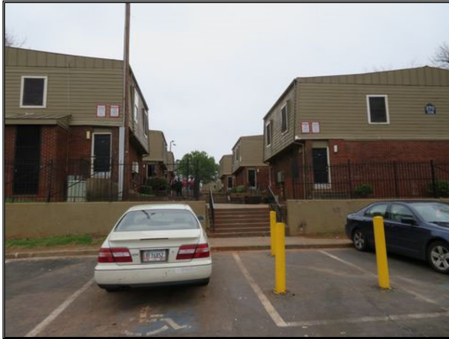
P53-Retaining Wall/Stair Sets
