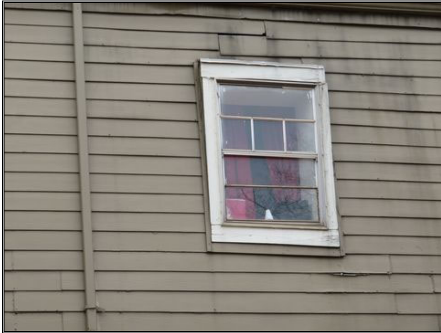
P55-Typical Window in Poor Condition
