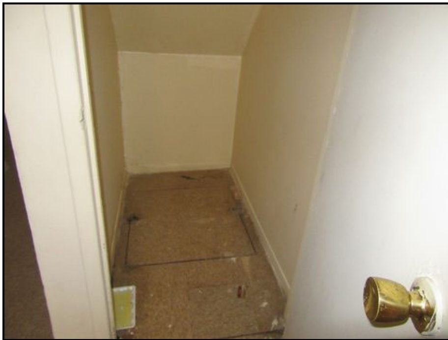
P76-Closet with Crawl Space Entry
