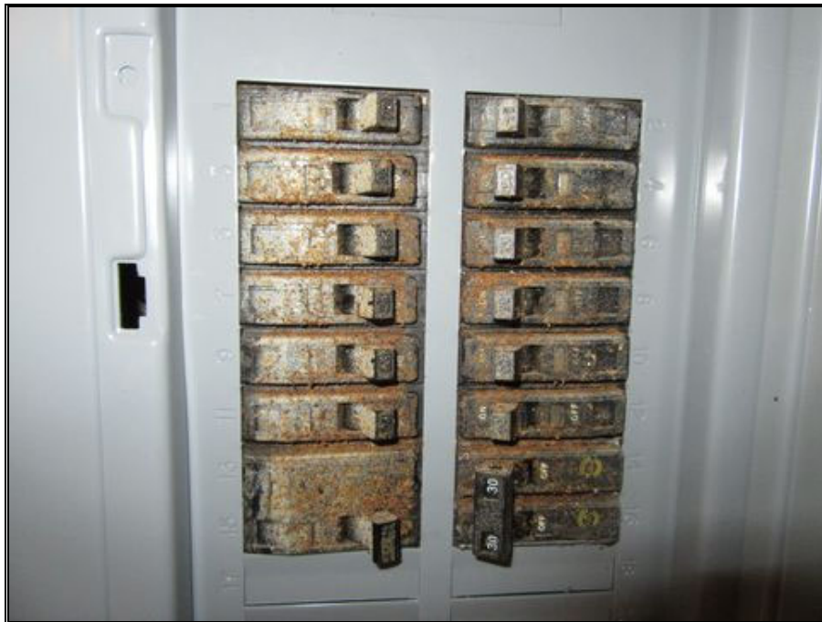
P80-Typical Apartment Panel Box
