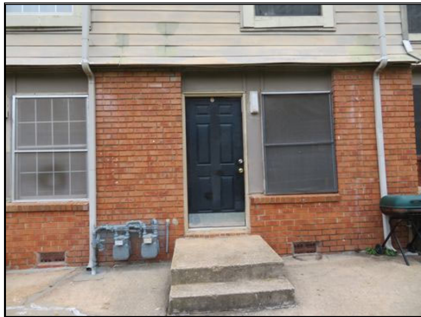
P94-Townhouse Entrance/Gas Meters
