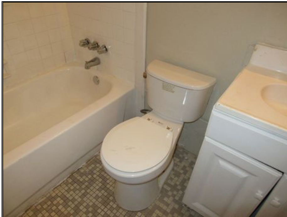
P72-Vacant Unit Bathroom
