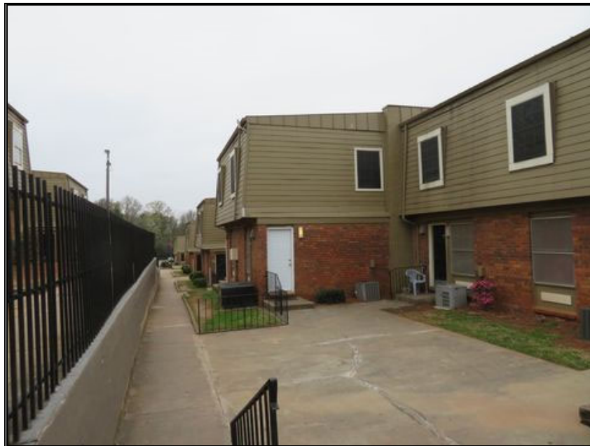
P96-Concrete Retaining Wall on North Side
