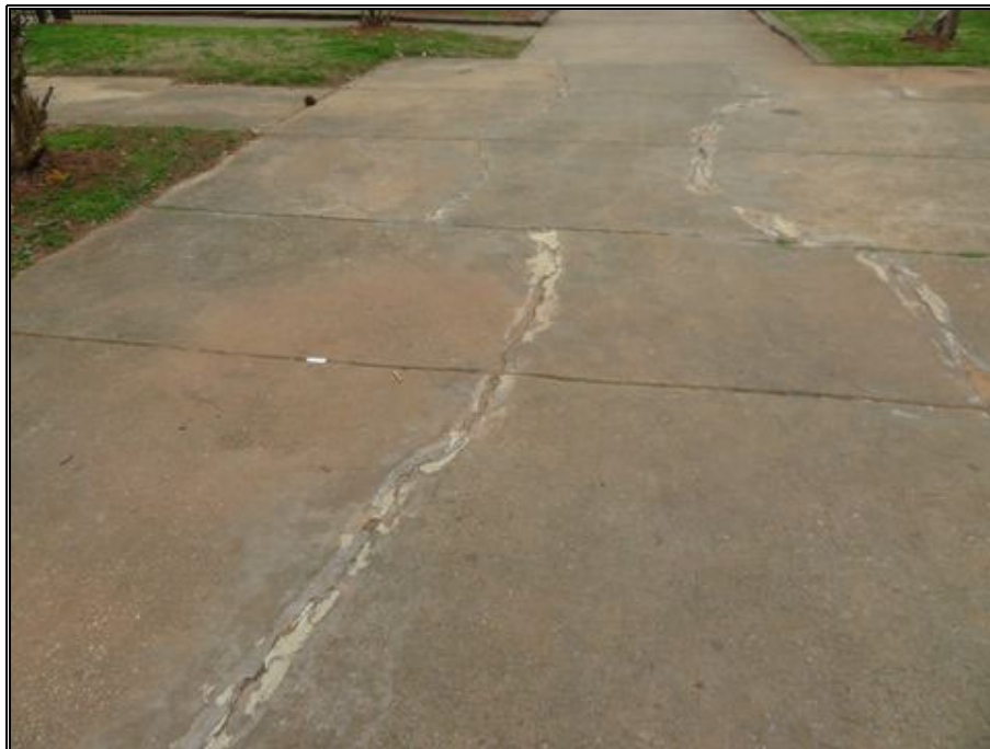
P46-Concrete Cracking
