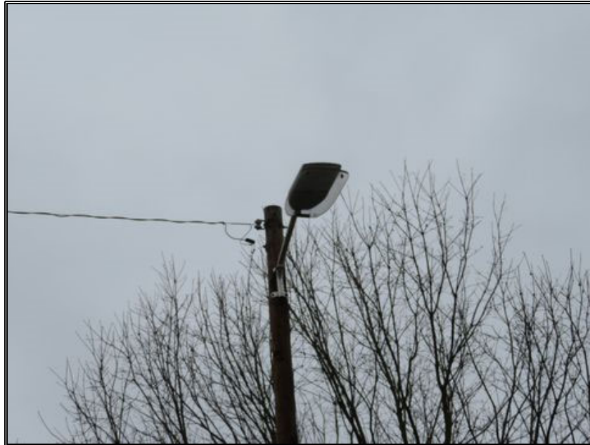
P95-Typical High Pole Light
