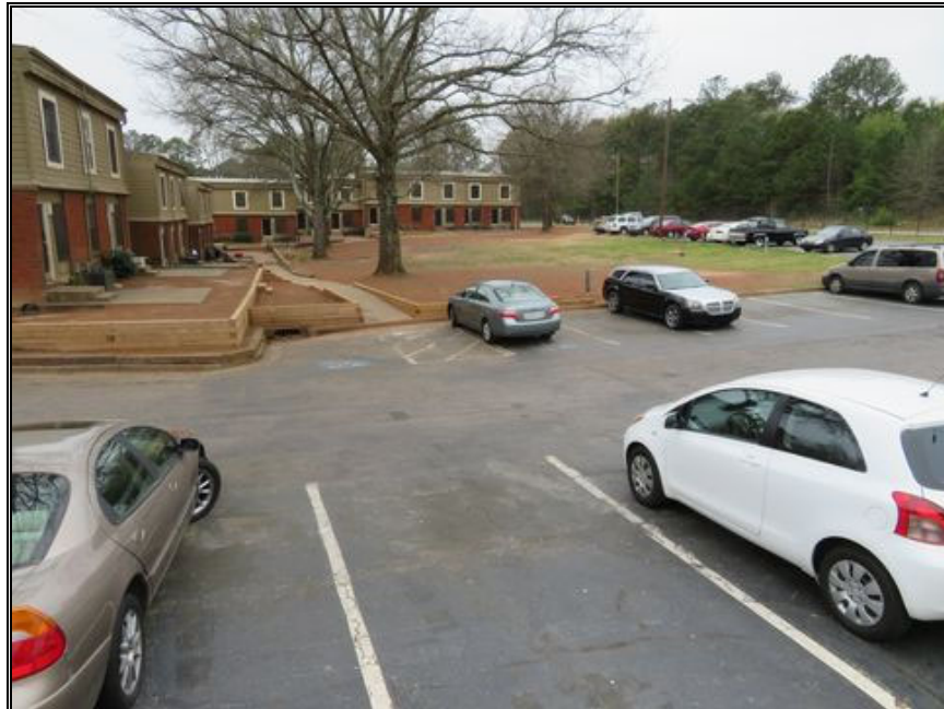
P56-South Section Parking Area
