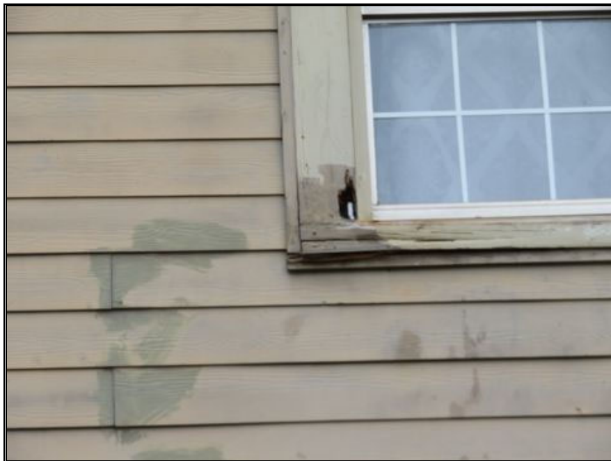
P20-Example of Dry Rot on Window Framing
