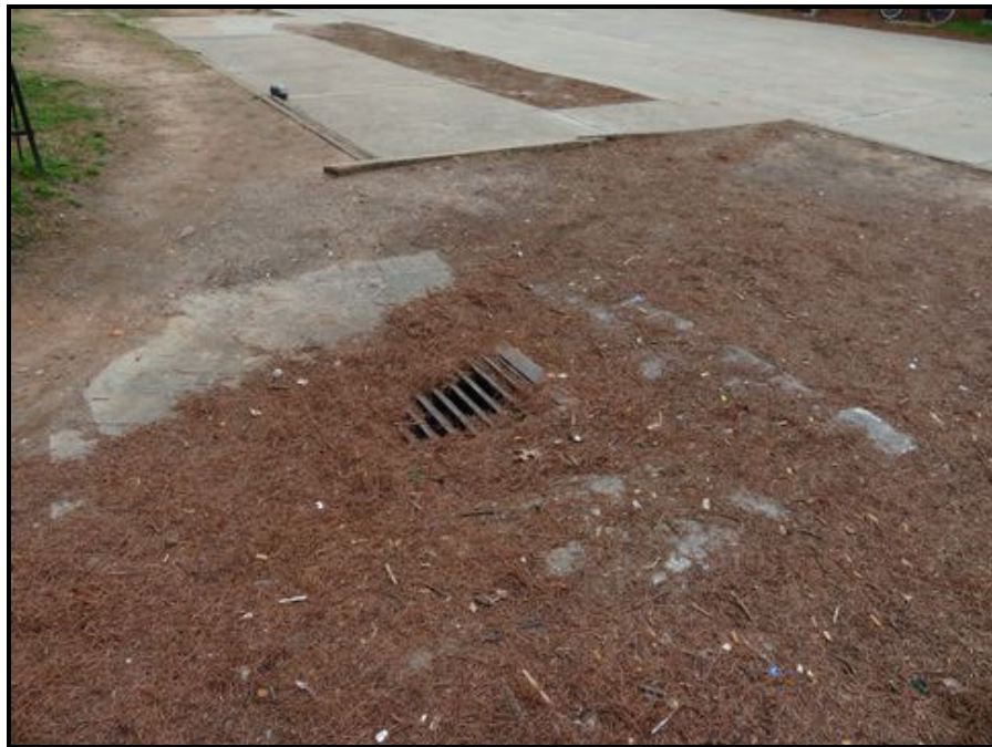
P28-Typical Yard Drain
