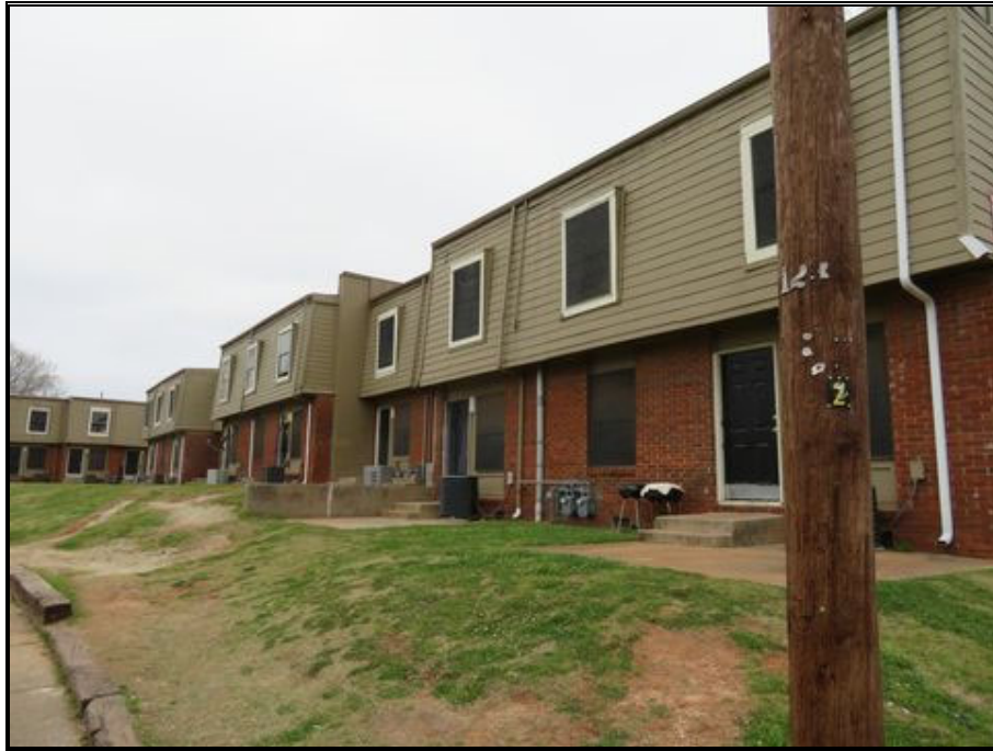
P33-14-unit Building Rear Elevation
