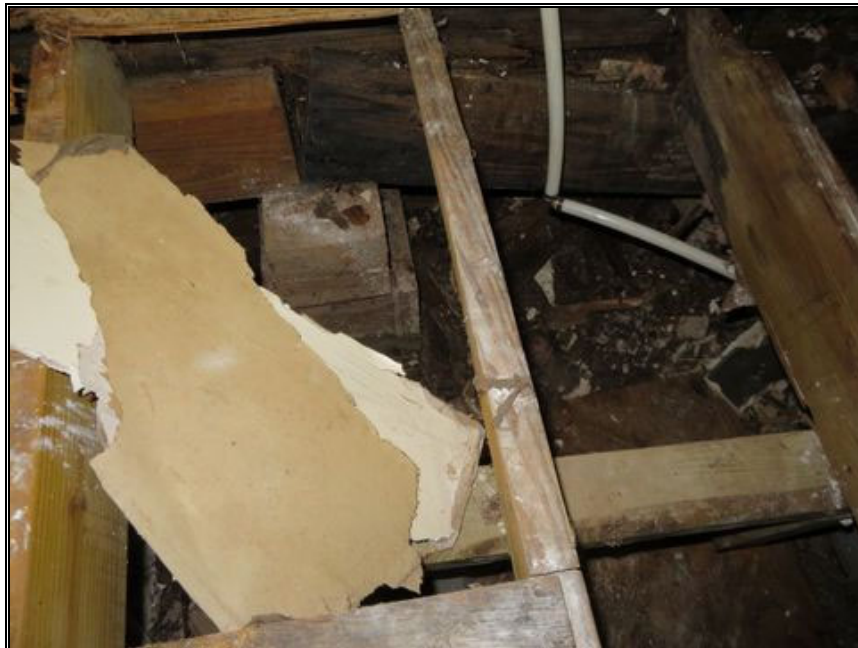
P30-View of Crawl Space
