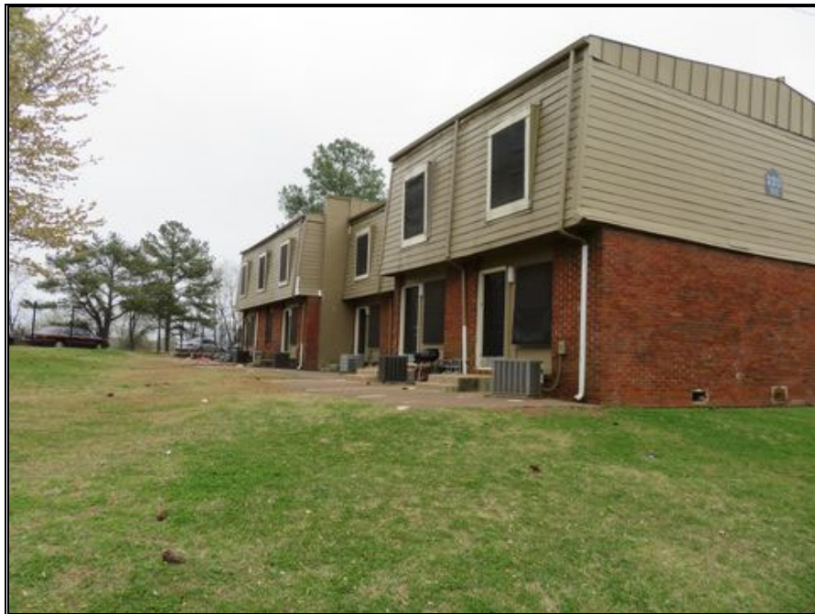
P48-Building (Fire Wall in Middle)
