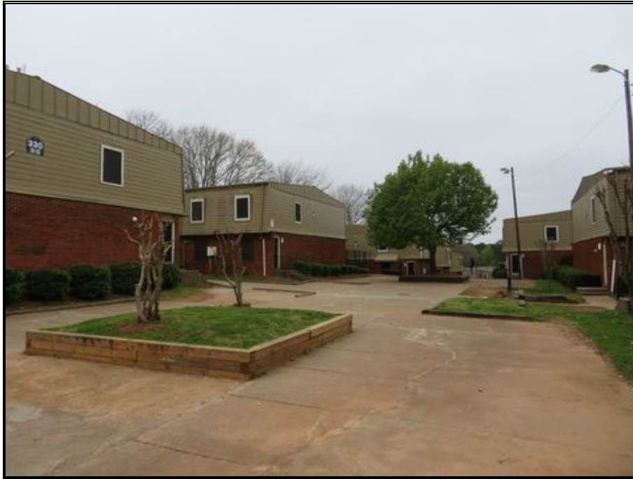
P47-Typical Courtyard Area (Former Parking Area)
