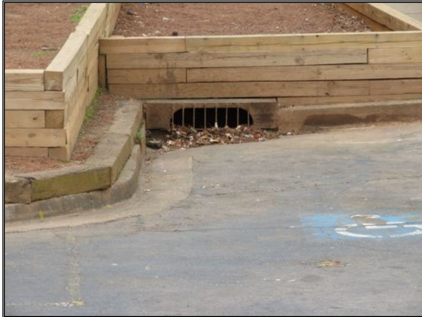
P57-New Wood Retaining Walls/Curb Drain
