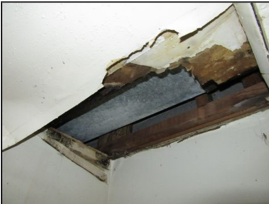
P92-Ceiling Water Damage
