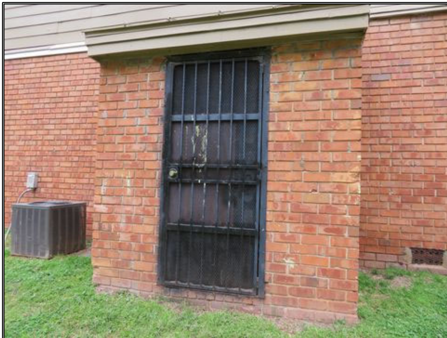
P12-Typical Electric Meter Room
