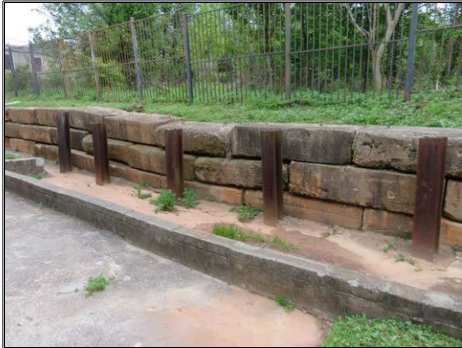
P9-Block Retaining Wall and Iron Fencing
