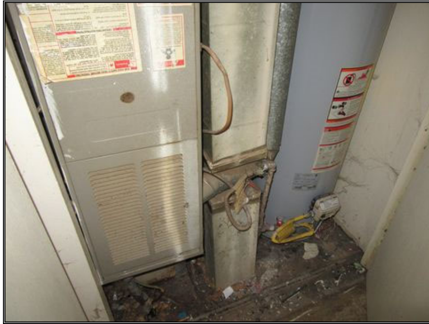
P65-Typical Furnace and Hot Water Tank
