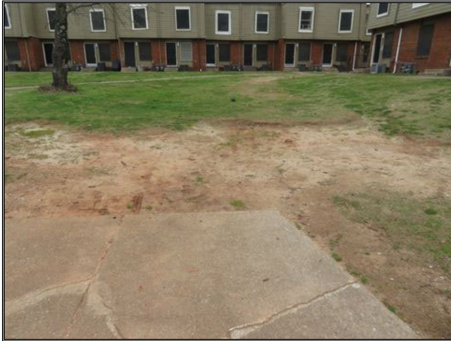
P43-Example of Erosion on the Property
