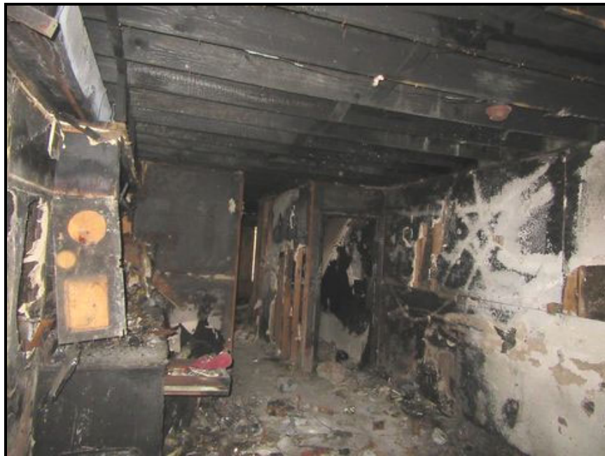
P88-Burned-Out Down Unit
